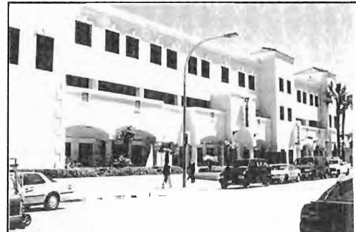
Screened parking structure.
