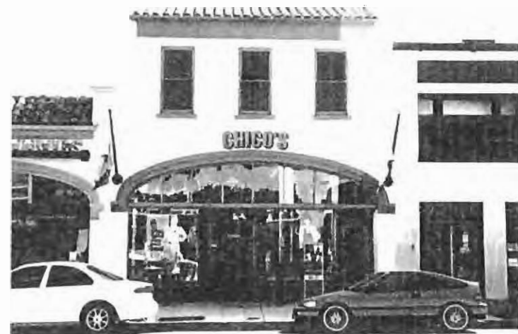
Placement of sign is appropriate.
