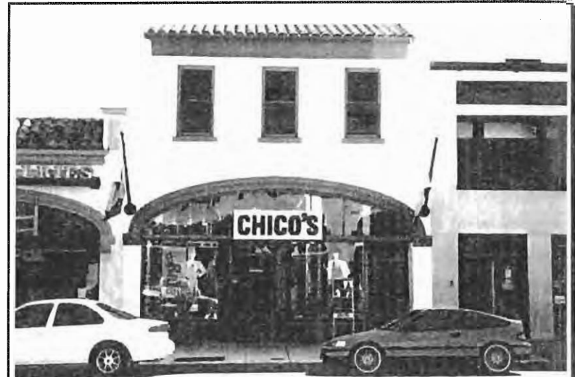
The sign is located in an inappropriate location.
